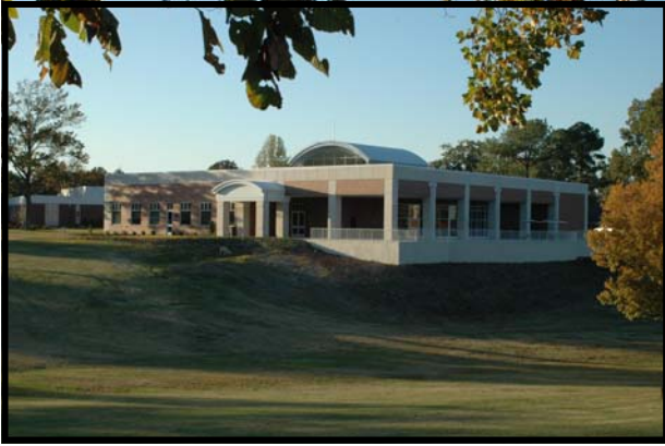
DSCC Dyersburg Campus Student Center
